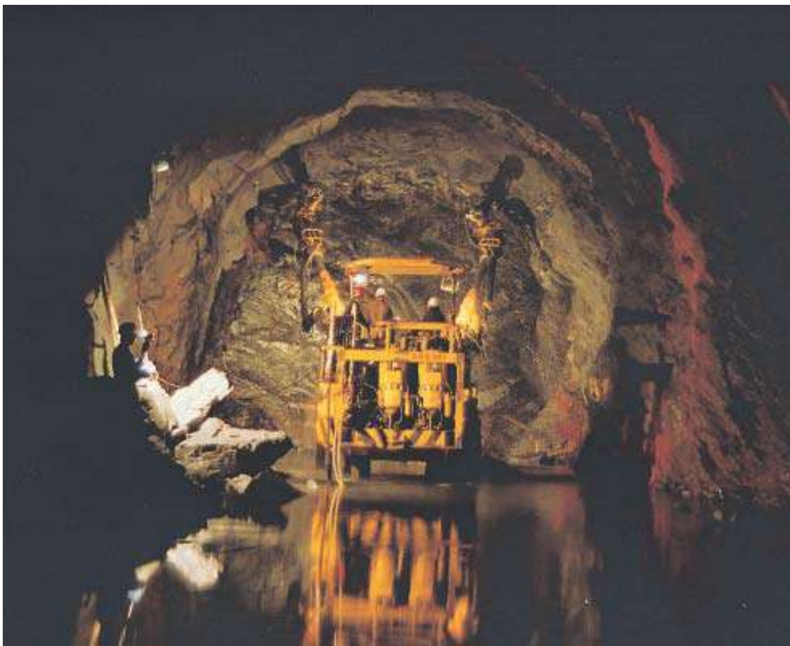
390 MW Dulhasti Project (J&K) - Adit Tunnel
