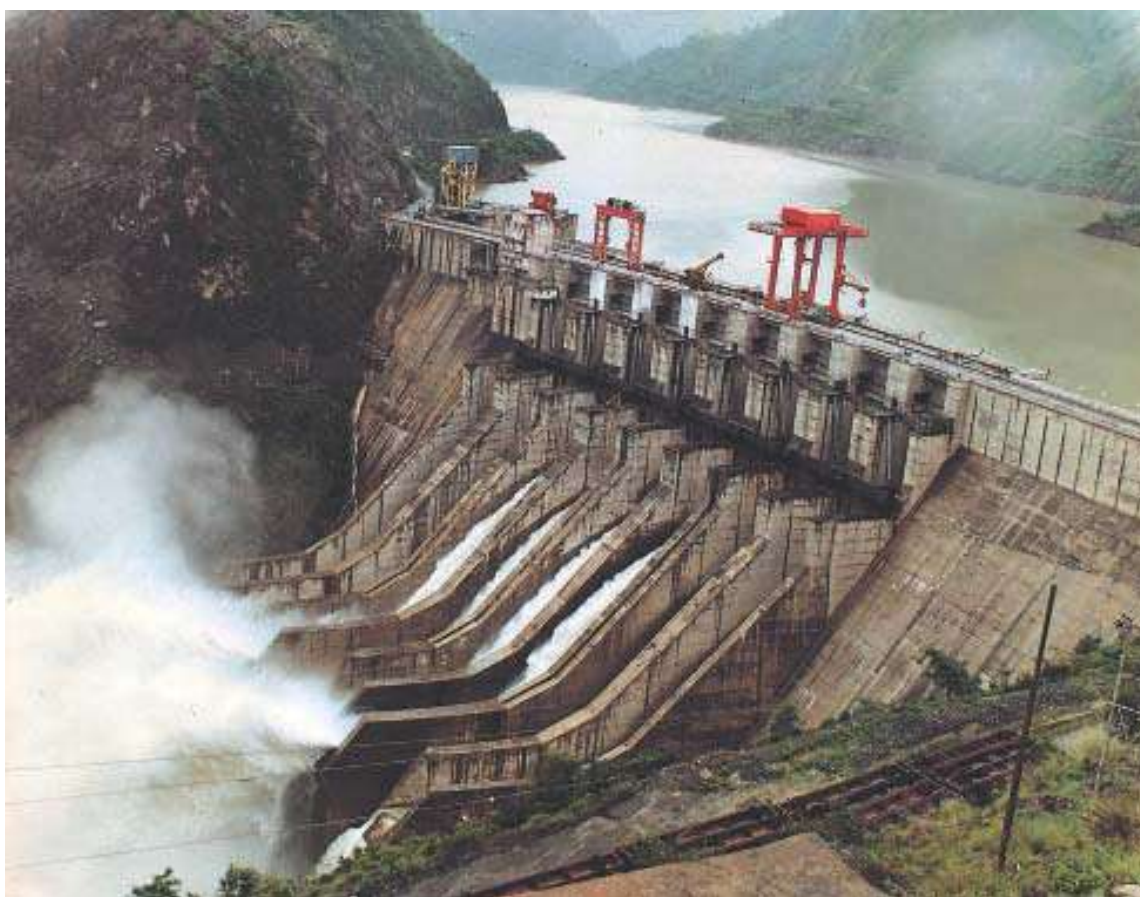
A view of Chamera Dam
