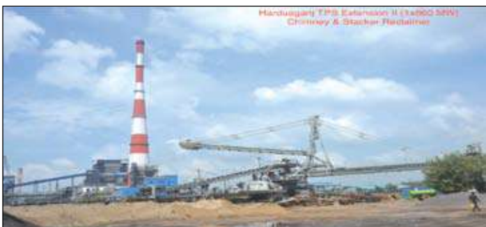
Harduaganj TPP Extn II (1x660 MW)-UP
