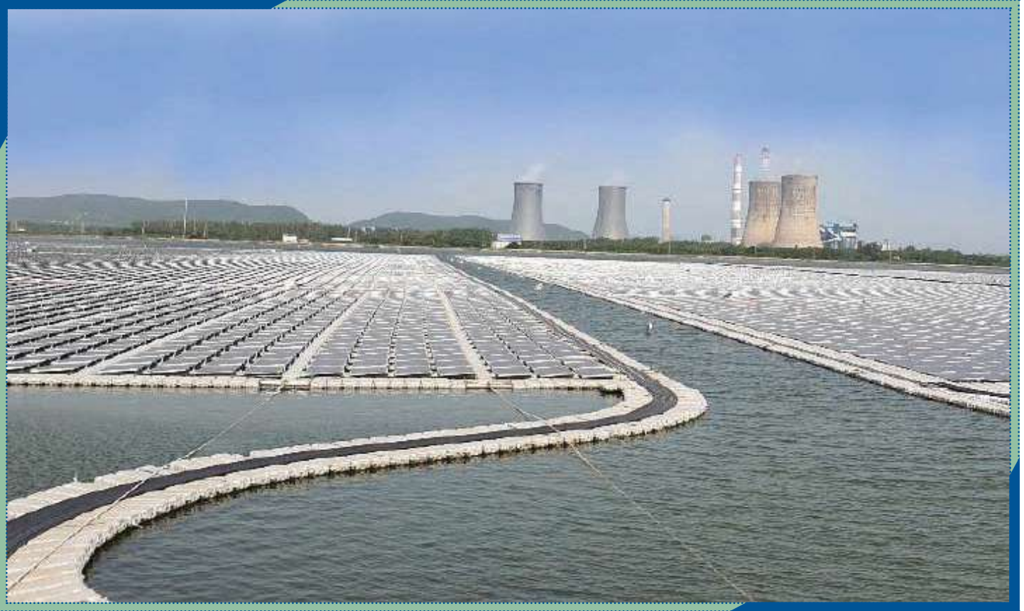
36 MW Floating Solar Project - Visakhapatnam, NTPC
