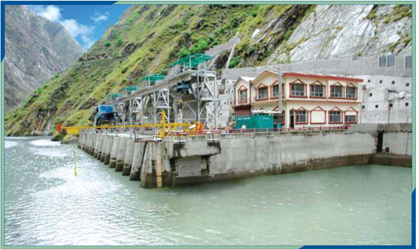
1500 MW Nathpa Jhakri Power Station
