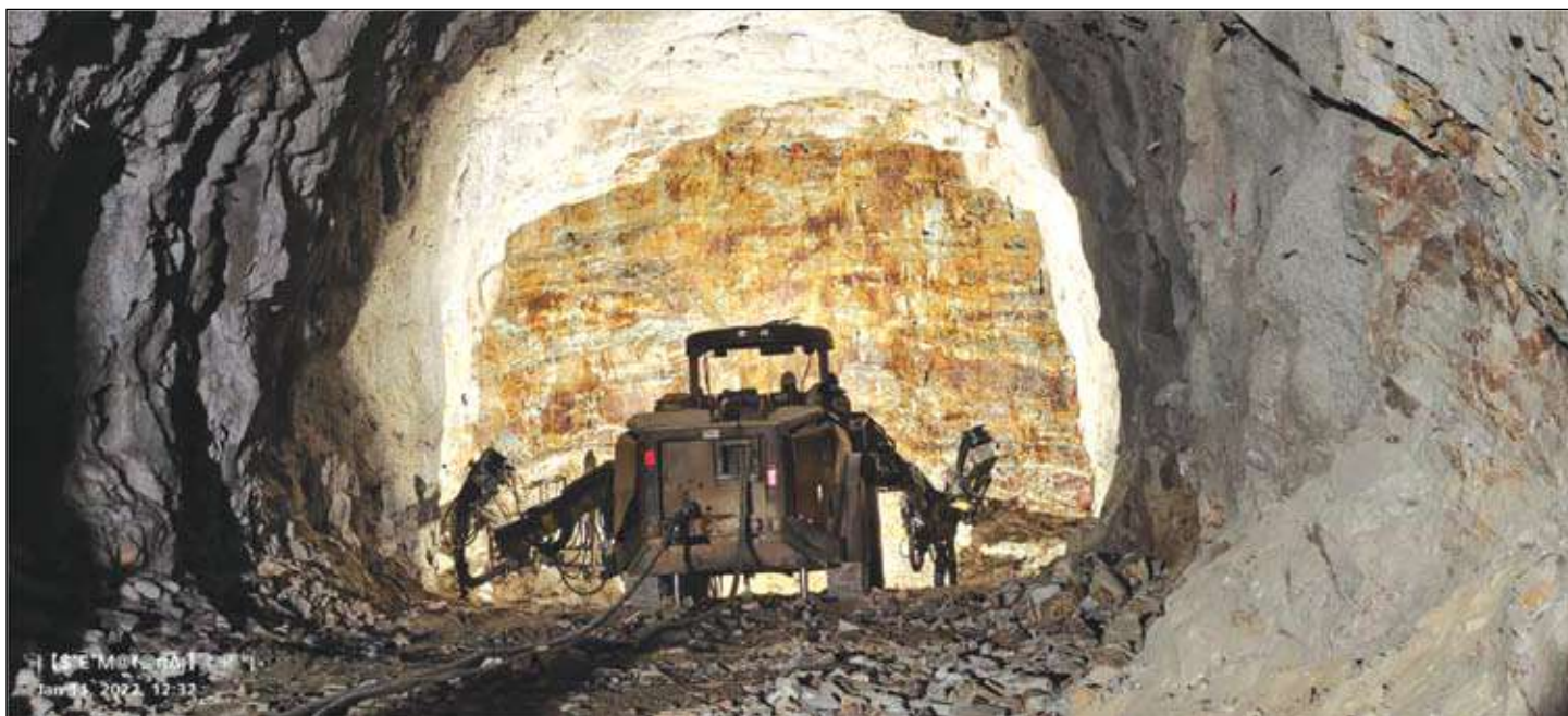
Hrt Excavation – Kiru H.E. Project
