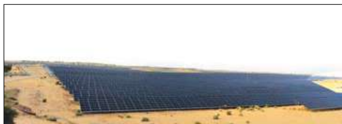
600 MW (900 MWp) India's Largest Solar PV Plant at Bikaner, Rajasthan funded by PFC.
