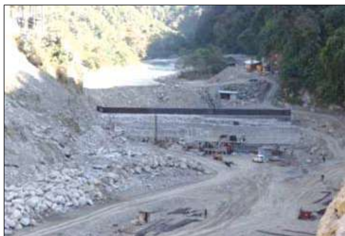
Arun-3 HEP (900 MW) - Coffer Dam Area Construct
