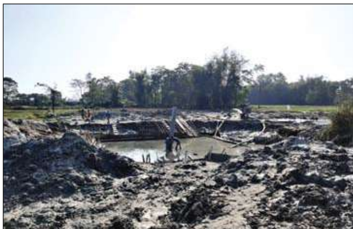
Fondation works in 400 kV Jigmeling - Alipurduar transmission line
