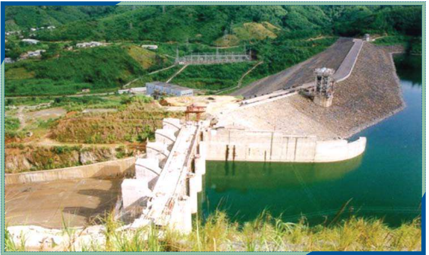
View of Dam & Power House of 75 MW Doyang Hydro Power Station, Nagaland
