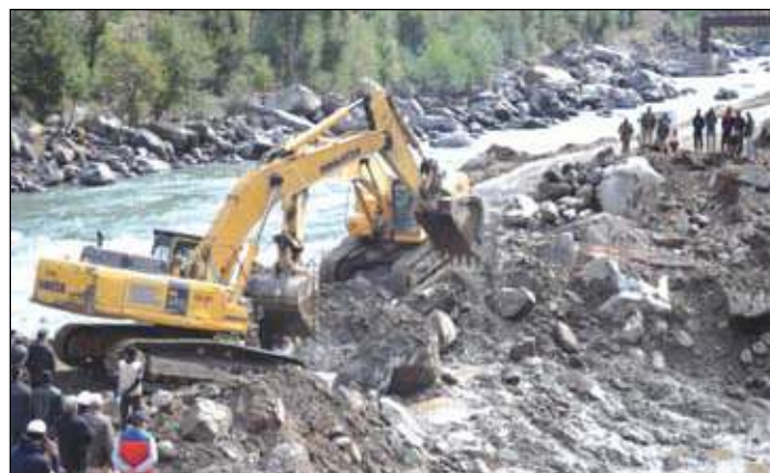
River Diversion - Pakal Dul H.E. Project
