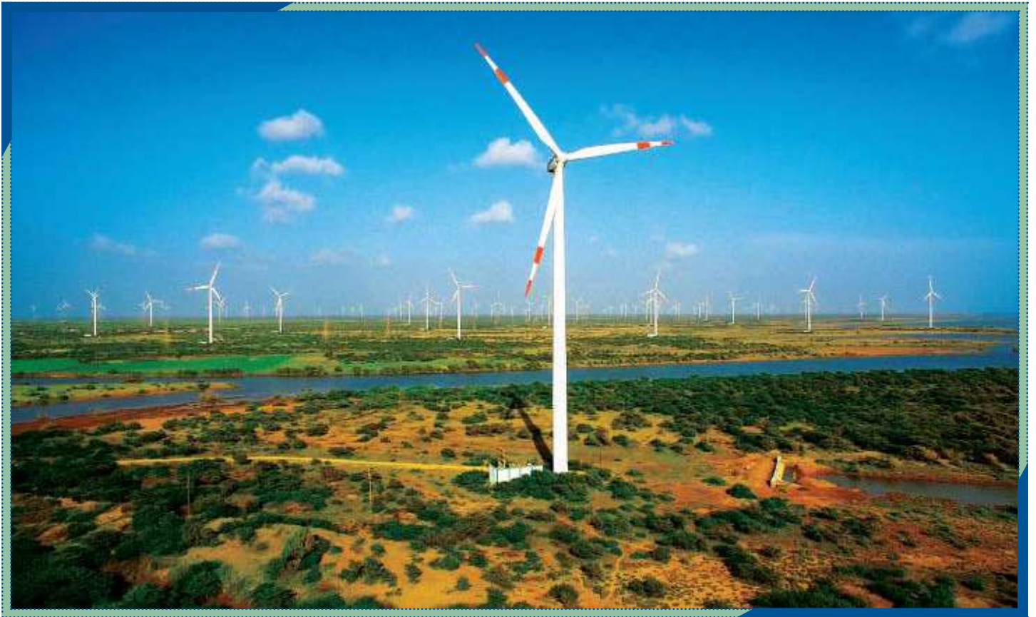
Suzlon wind farm, Bhuj, Gujarat
