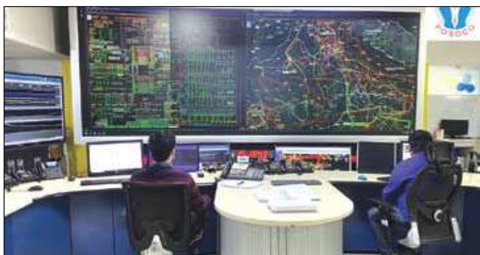
National Load Despatch Centre Control Room
