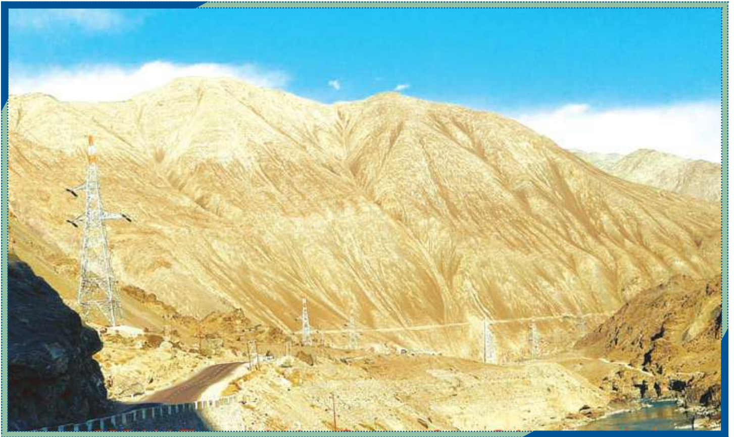
220 kV Transmission system from Srinagar to Leh
