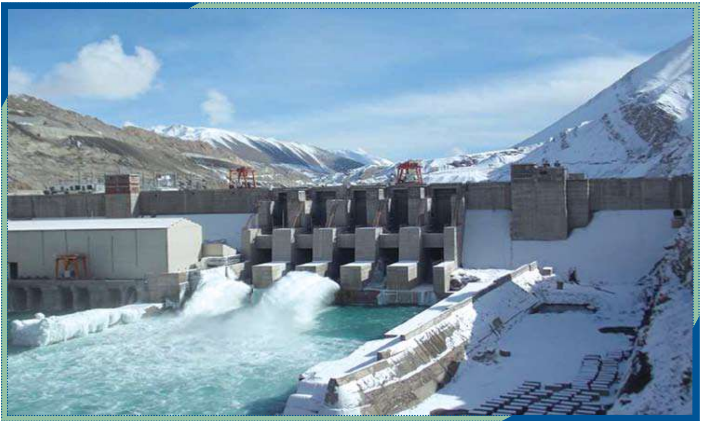
45 MW Nimoo Bazgo Power Station
