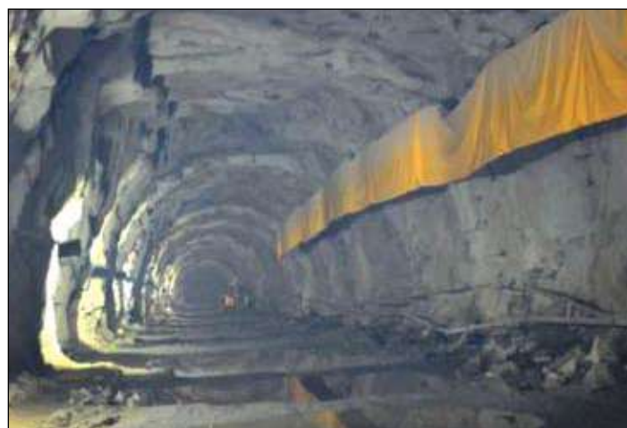
Luhri Stage-1 HEP (210 MW) - Diversion Tunnel Construction
