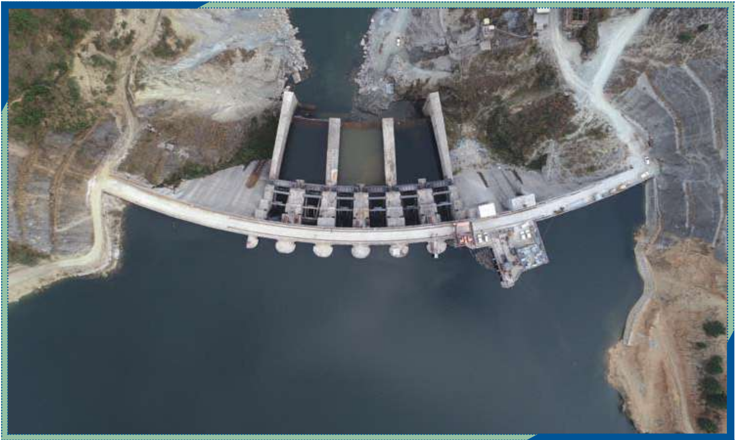
Aerial view of Bichom Dam of recently commissioned 600 MW Kameng Hydro Power Station, Arunachal Pradesh
