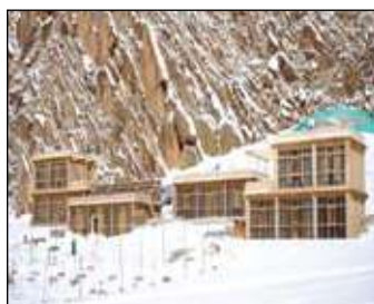
Passive Solar Heated (PSH) Buildings of HIAL
