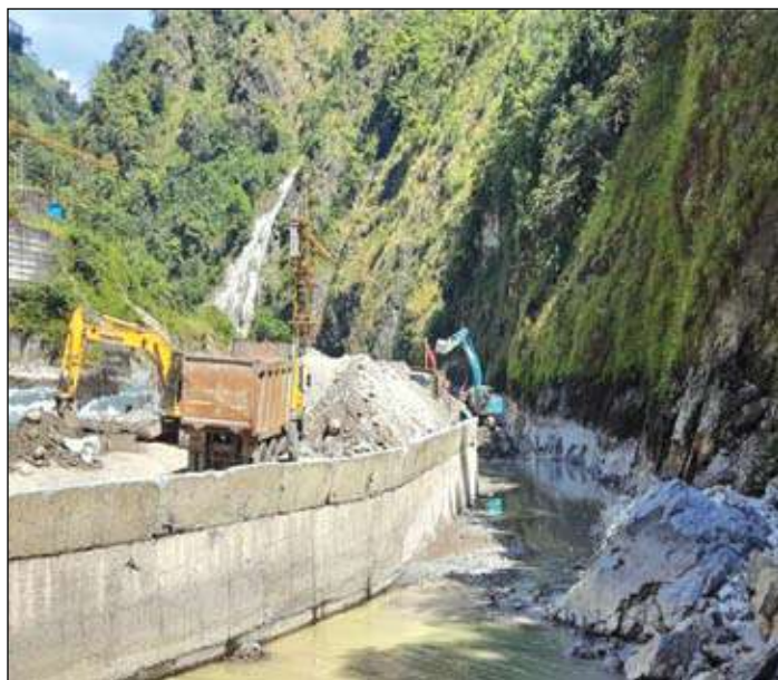
River Diversion - Rangit-IV H.E. Project
