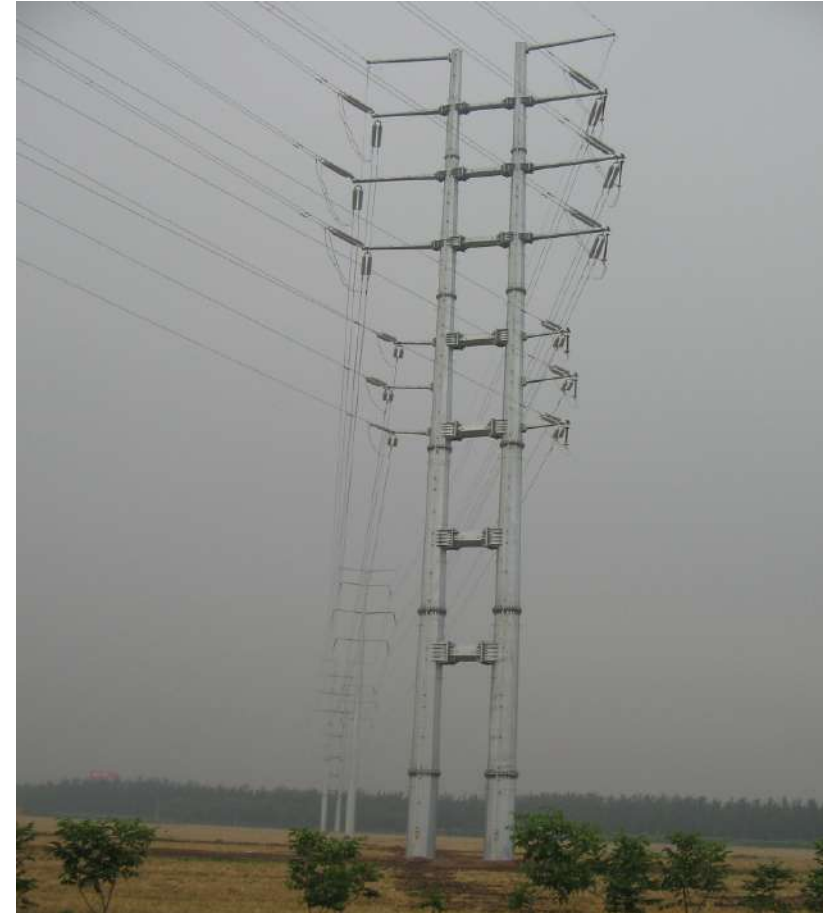
(B) MONOPOLE WITH MULTI CKT & MULTI VOLTAGE
