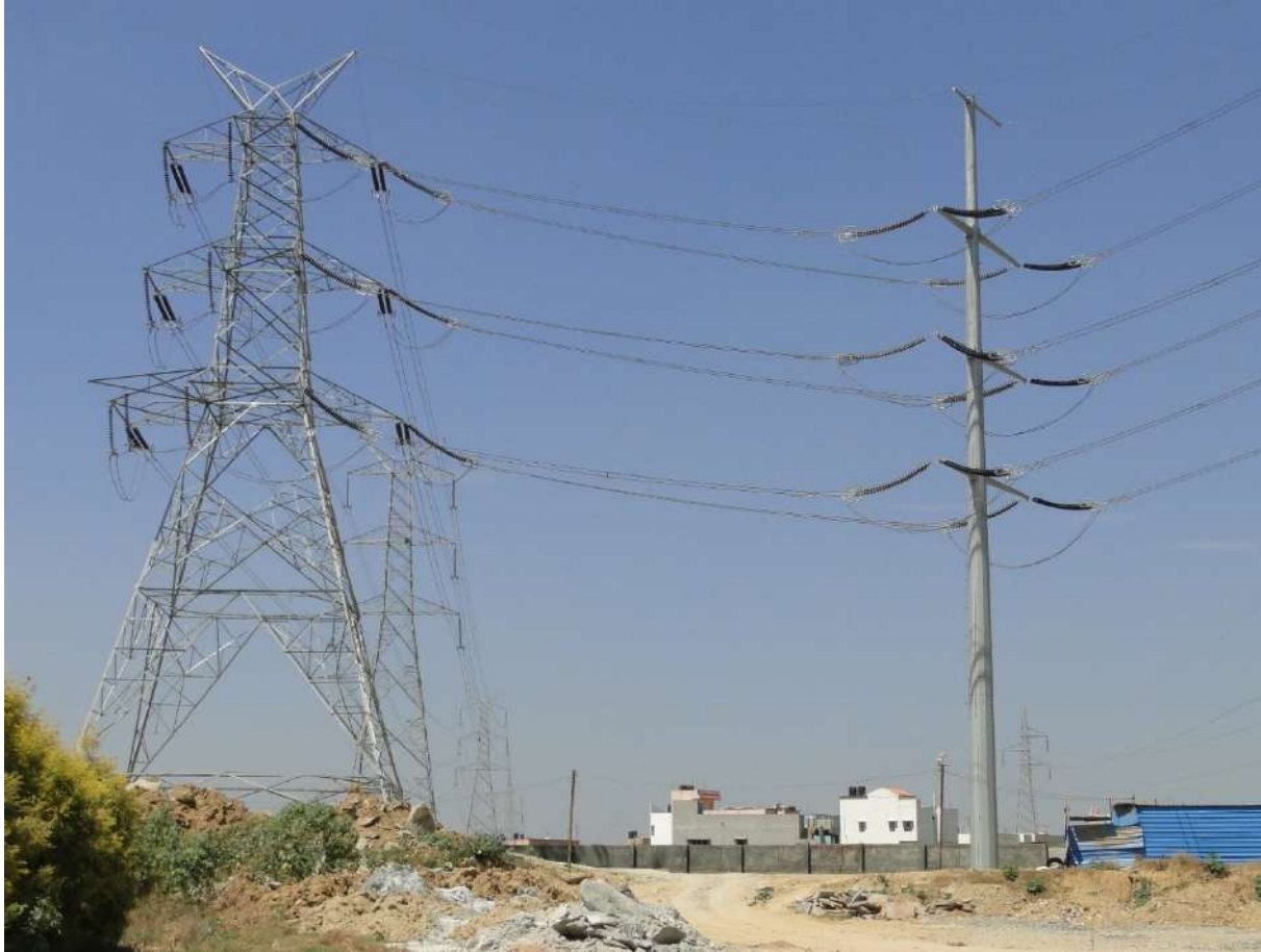
(A) LATTICE AND MONOPOLE STRUCTURE
